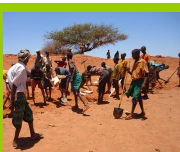
Cash-for-work in action – excavation of water catchment, Lower Shabelle
